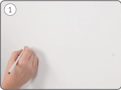
Using the wall mounting dimensions and a spirit or laser level, measure and mark the L1 size for your specific Glass Panel Heater on the wall. This varies depending on your heater size.
