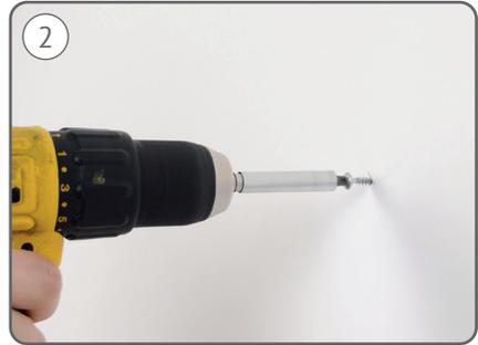
Drill holes into the wall and drive fixing screws into place. Use suitable fixings for your wall type. Leave approximately 5mm of thread visible.
