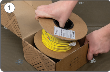
1 Remove your heating cable from the box and take off the card protection sleeve.
