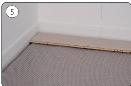
5 Follow the manufacturer's instructions to lay the engineered timber flooring.
