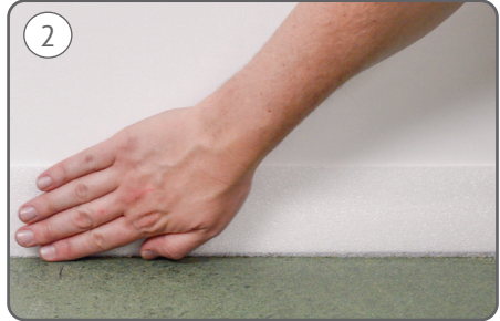
2 Fix perimeter foam around the edge of the room using the self-adhesive strip or staples.
