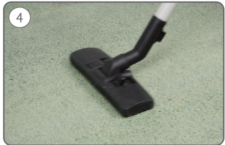
4 Ensure the substrate is clean and free from any dust and debris.
