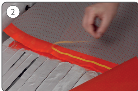
2 Stick parallel runs together using the self adhesive strip on each run of overlay.
